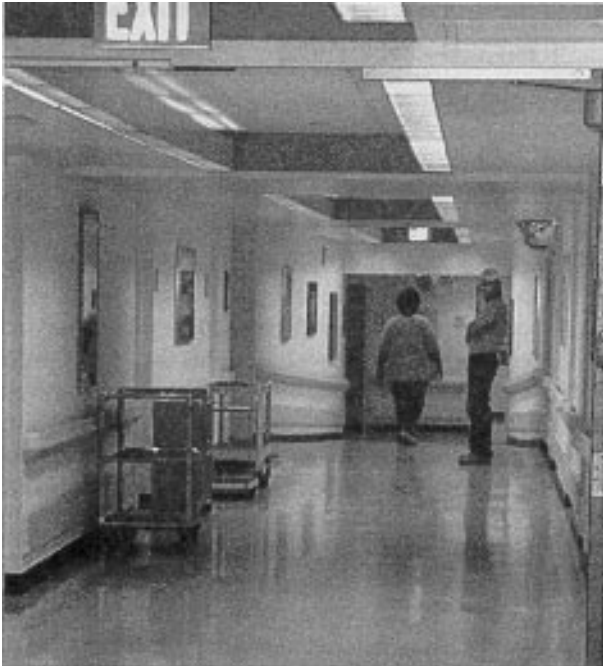
Figure 7-3—Corridor lighting, using linear fixtures, after remodeling
